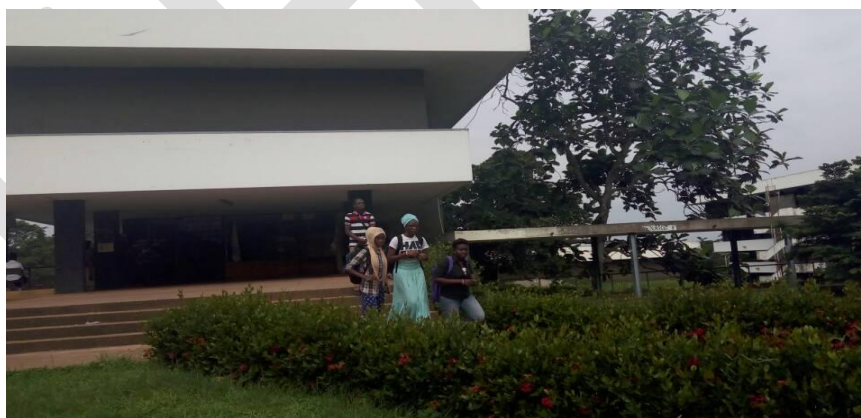
Figure 10. A section of the Humanities Block, Obafemi Awólówo University, more than 50 years after Lasekan painted the movement into Ife. Photograph by Stephen Fọlárànmí, 2017
