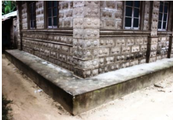
Fig xii view showing external skirting differentiating two pointing techniques at window sill (Author 2016)
