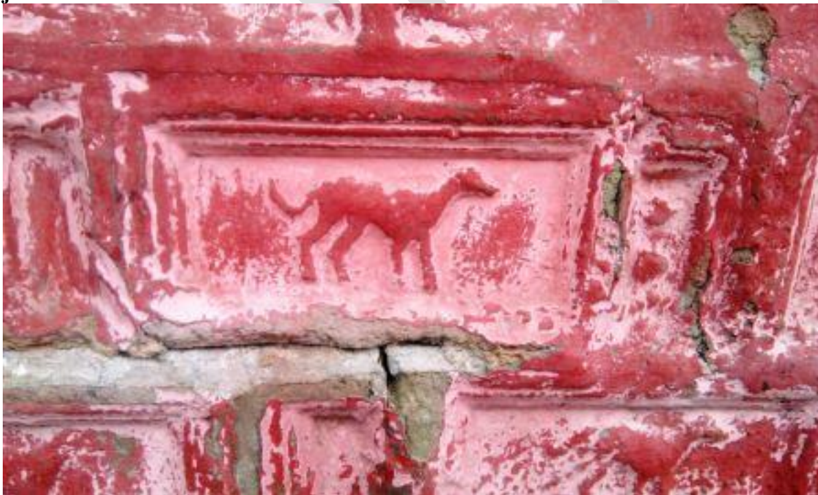
Fig vii detail of relief ornamentation on finished concrete block depicting a hunting dog (Author 2016)
