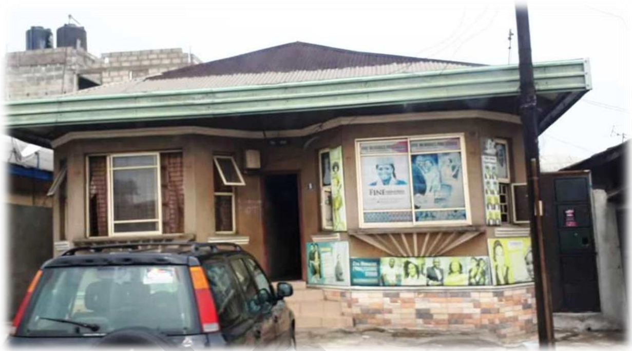
Fig xx The late-model showing symmetrical three-sided front (This sample shows some recent renovations such as sliding windows in place of the original wooden shutters with jalousies) Author 2019
