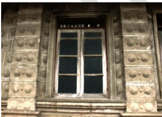
Fig x casement window with glass pane used in place of wooden shutters (Author 2016)
